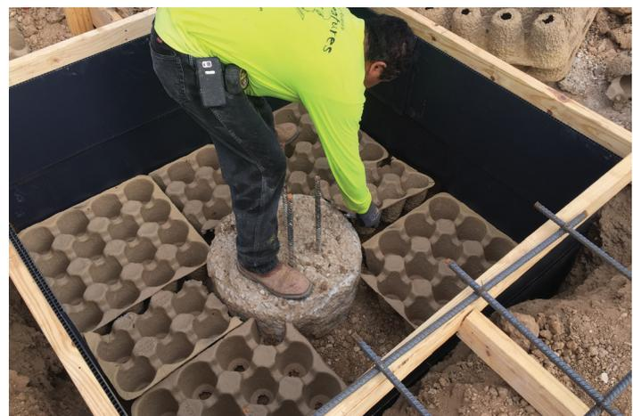
America’s reliable void form, Reliable Molded Pulp Voids™
